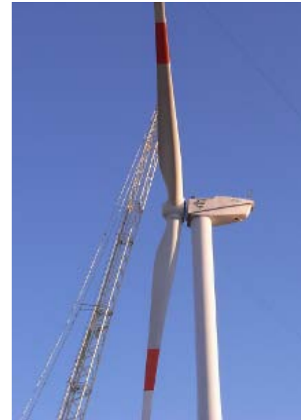
December 20, 2007, REpower North 2MW Wind Turbine was installed successfully
