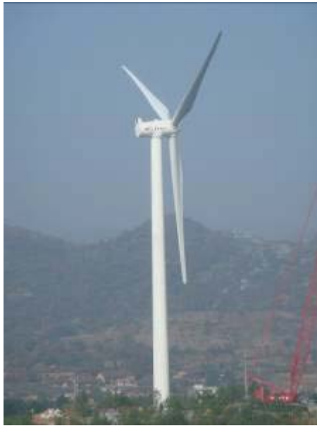
November 2007, CSR Times 1.65MW Wind Turbine successfully integrated into grid
