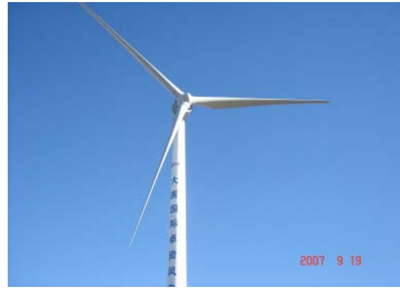
September 19, 2007, XEMC 2MW wind turbine in Datang wind farm
